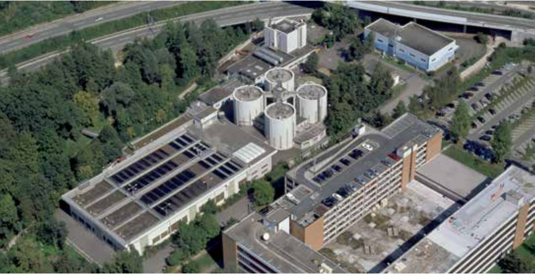
NEUGUT WWTP (150,000 PE)
